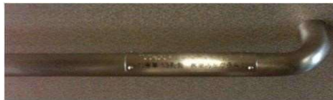
Handrail with Braille Information Panel
